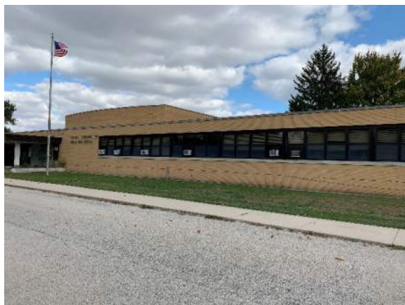
Photo A02 – West Elevation
