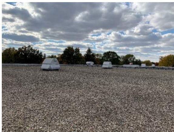
Photo A17 – Gymnasium Roof (Upper)
