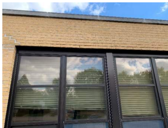
Photo A13 – Tuckpointing, Typical
