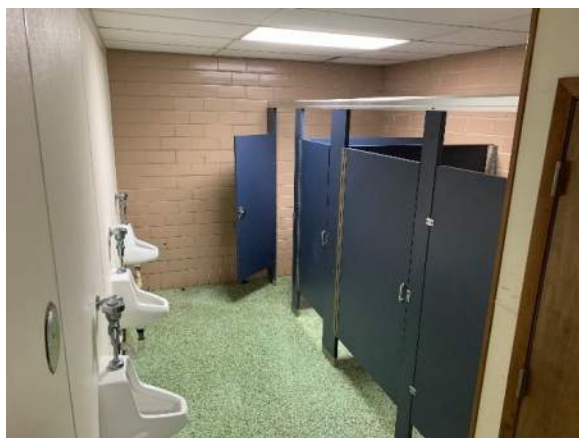
Photo A06 – Typical Restroom
