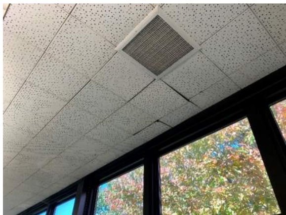
Photo A20 – Asbestos Ceiling Tile
