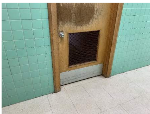
Photo A04 – Corridor Door w/ Grill
