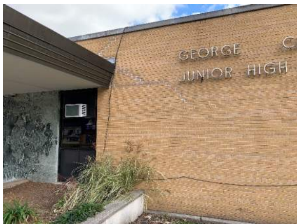
Photo A12 – Tuckpointing at West Elevation
