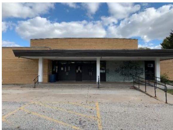
Photo A_C – Main Entry (Exterior)
