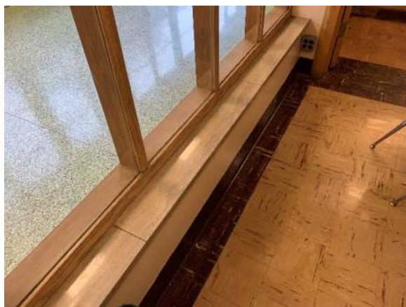
Photo A18 – Terrazzo & Asbestos Floor Tile
