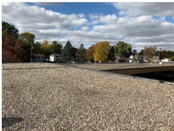
Photo A16 – New/Old Roof (Lower)
