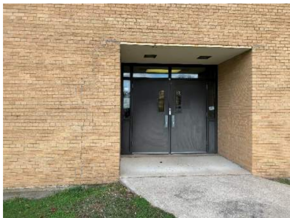
Photo A14 – Masonry Repair, East Elevation
