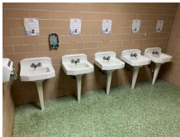
Photo A07 – Typical Restroom
