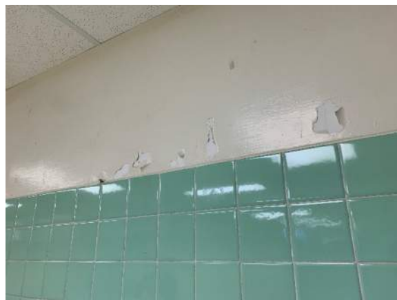
Photo A21 – Painted Finish (at Corridor)
