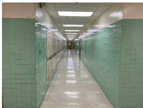
Photo A05 – Dead End Corridor
