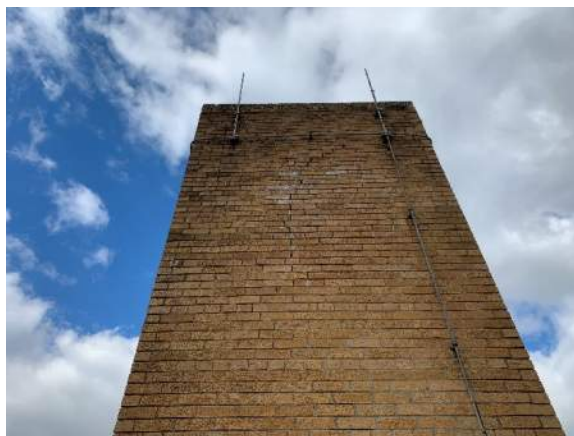
Photo A15 – Masonry Repair, Chimney
